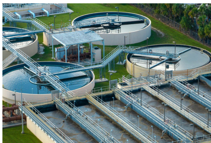
Figure 1. Wastewater treatment plant – biosolids source
