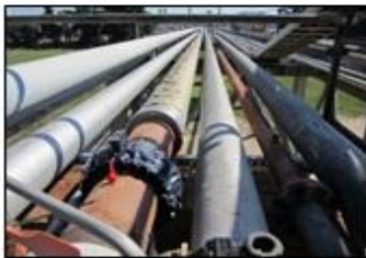
Probe Collar in position
