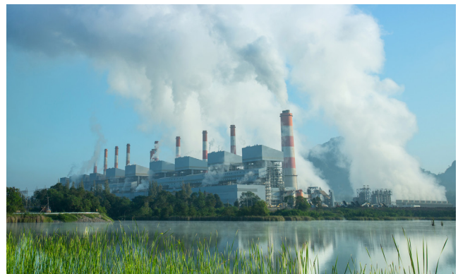
Coal-fired power plants: largest anthropogenic Hg source.
