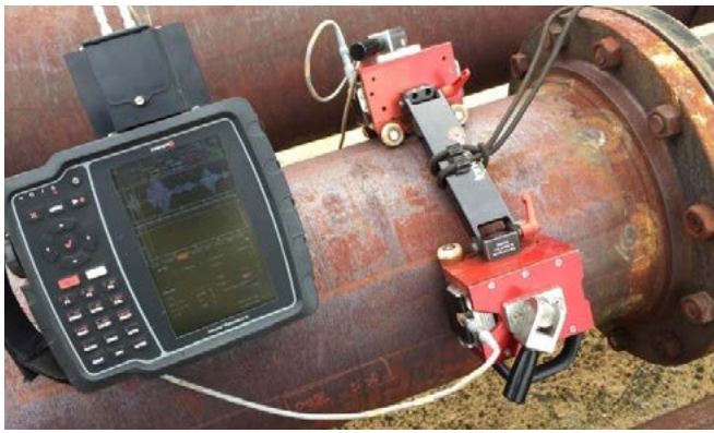
MRUT-A Mode scanner on a 12" pipe
